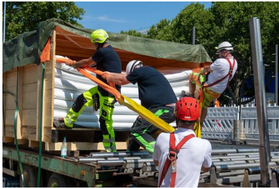
Figure 6: Preparation of liner for pulling process
