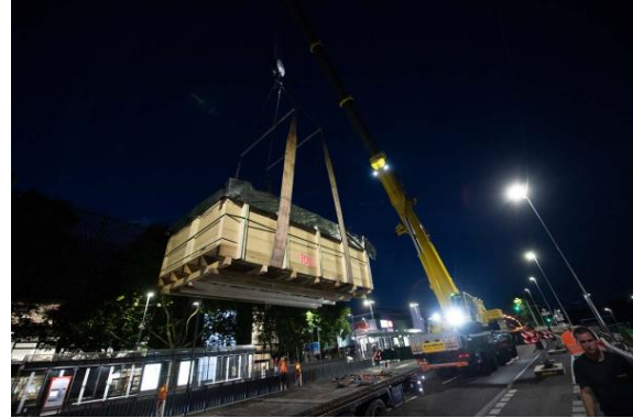
Figure 4: Handling of large dimension liner at the job site
