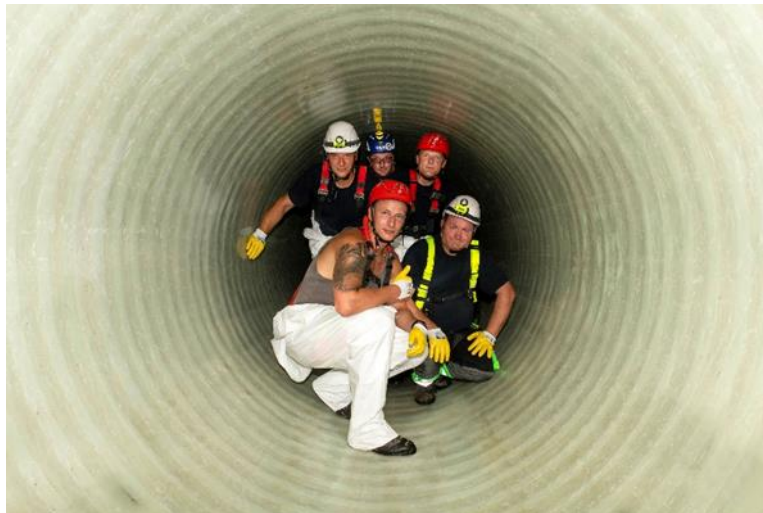
Figure 12: Members of the crew inside of the cured Alphaliner DN 1750
