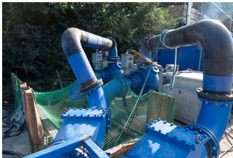
Figure 5: By-pass system with redundant design
